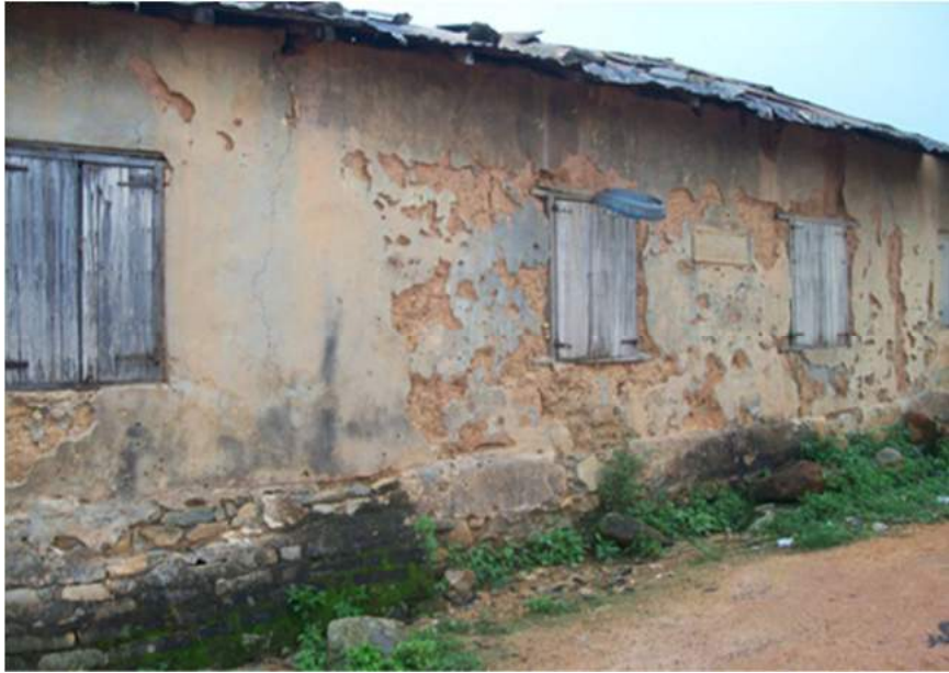
Plate 5: One of several ancient European styled houses constructed with stone blocks / bricks.
